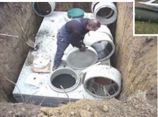
Replacing a septic tank and drain field
