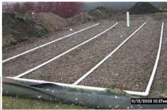
Replacing a septic tank and drain field
