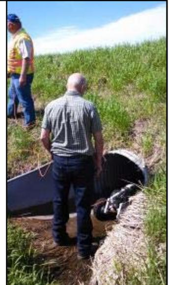
A culvert rover takes high resolution video of the inside of culverts.
